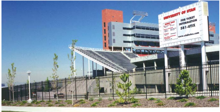
Mountain States Fence installed the stylish ornamental aluminum fence at the 2002 Olympic Plaza site at Rice-Eccles Stadium at the University of Utah.
